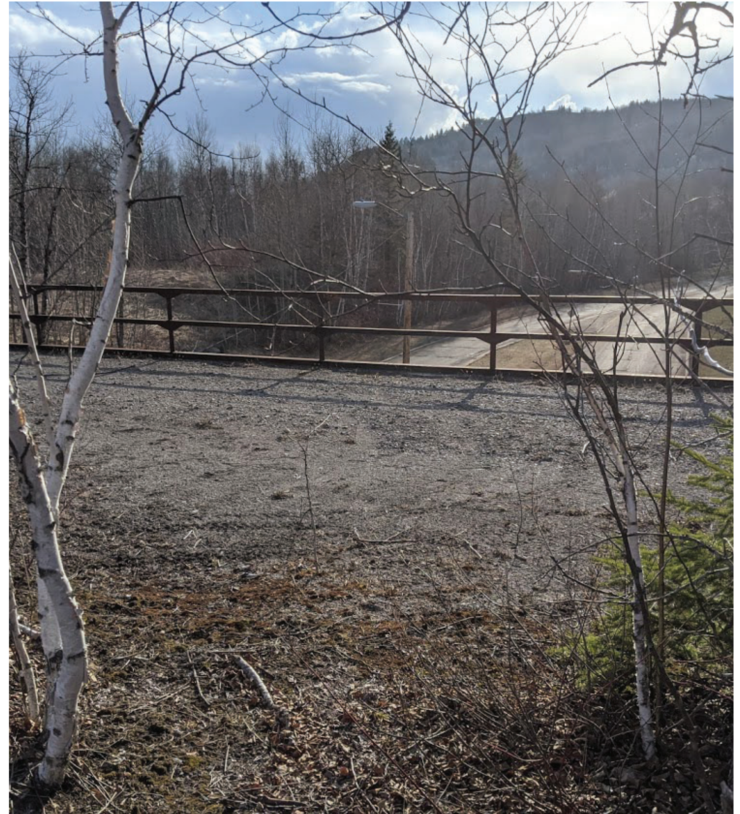
Railroad Bridge over 88th Ave W. near Morgan Park, 2020, Samuel Geer
