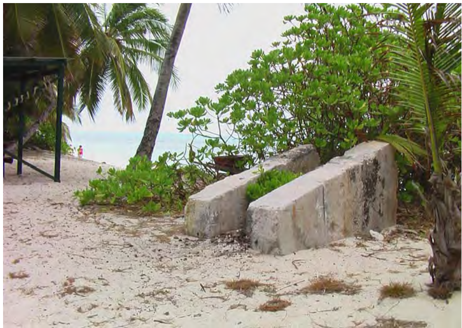
Slipway concrete plinth
