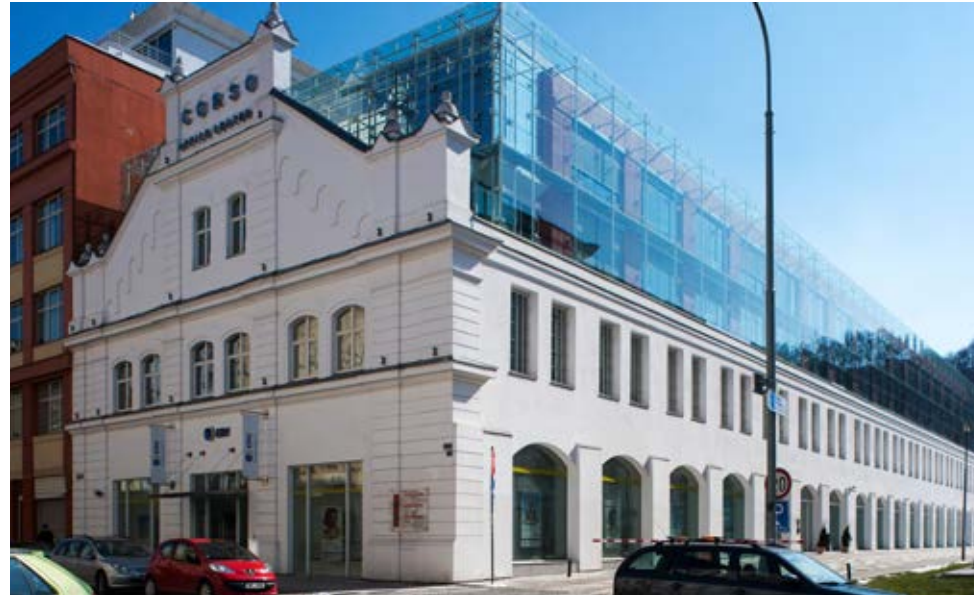
Corso building Karlin District, Prague
