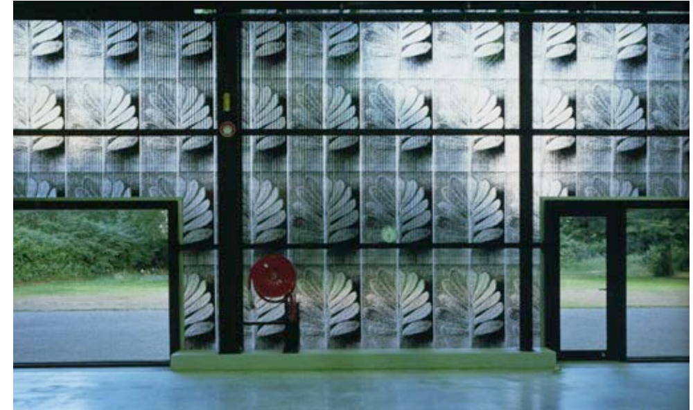
Motif hinting at history of business in natural, plant-based products Ricola storage building, Laufen, Switzerland
