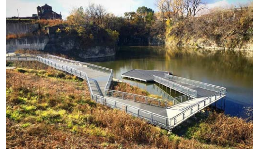
Reintroduced habitat at former quarry Palmisano Park, Chicago, IL
